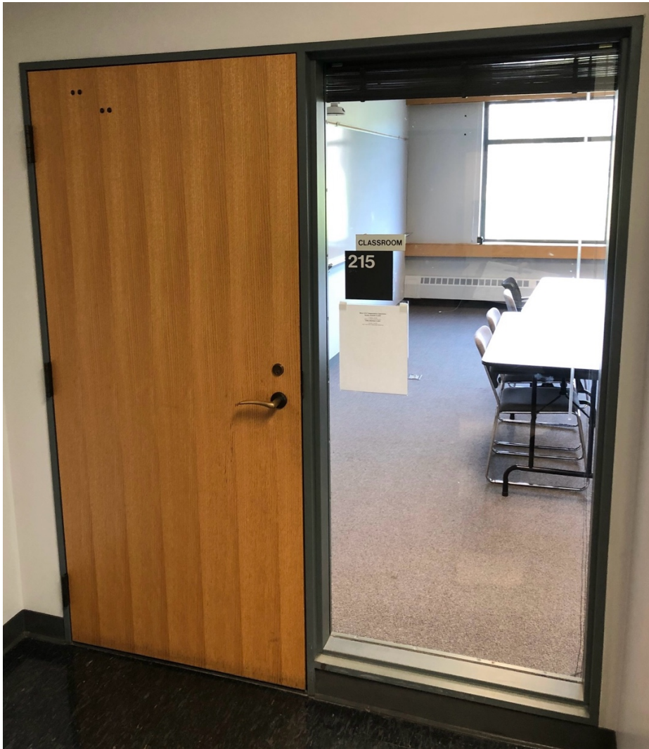
EXISTING DOOR AT CORRIDOR
