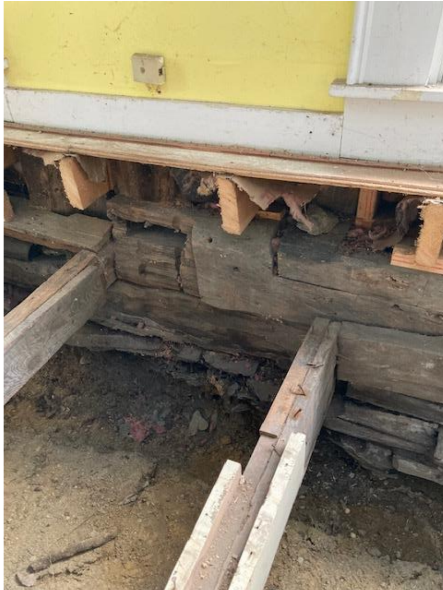
Granger Wing: sill and joist problems, south wall
