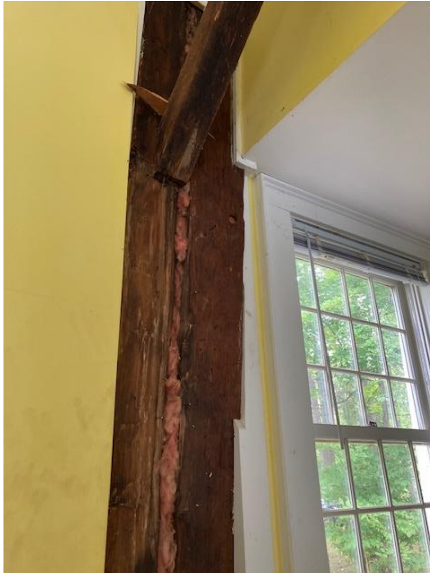
Granger Wing: out of plumb timber post and tapered window trim, north wall.
