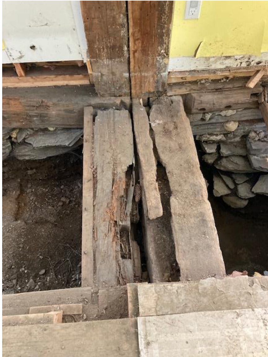
Granger Wing: Paired post and floor beams (sills) at 2 additions, south wall
