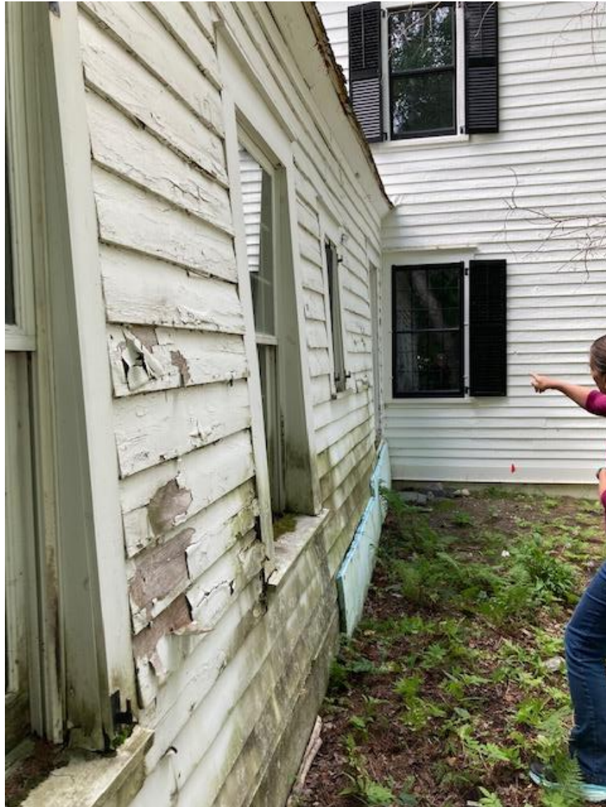
Granger Wing, north, clapboard and out of plumb wall
