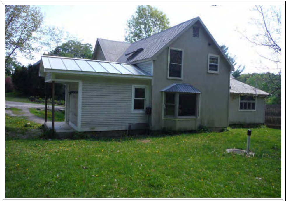
Additional Rear View
